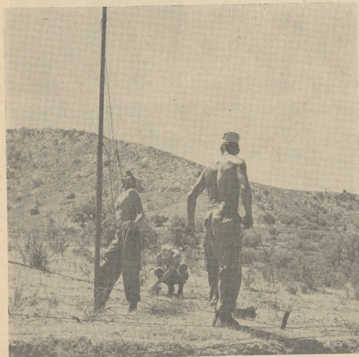
COMMUNICATIONS A MUST: It is hot dirty work but a lineman's job has never been easy. Weather or combat does not affect his aim to maintain communications. This Canadian crew is seen re-wiring over 130 miles of telephone cable. L. to R. they are: Pte P.V. Johnson, Cpl. R.L. Davis and Pte R.A. Oakley.
