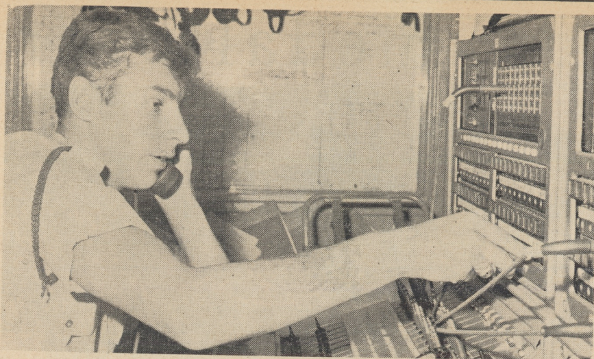
Sigm Sylvester of 644 Signal Troop connecting a subscriber to a required extension on the HQ Unficyp Exchange.
